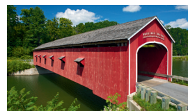
K505 Covered Bridge
